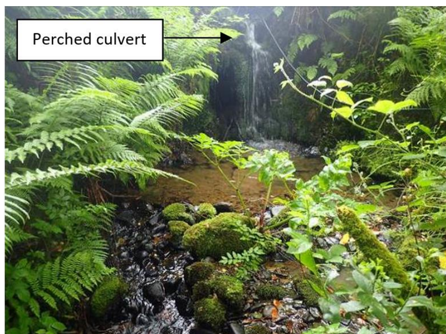
Plate 8. A perched culvert that likely limits the upstream passage of trout located at Site 2 on the 1 st Order Glennagross Stream, a tributary of the Crompaun Stream.
