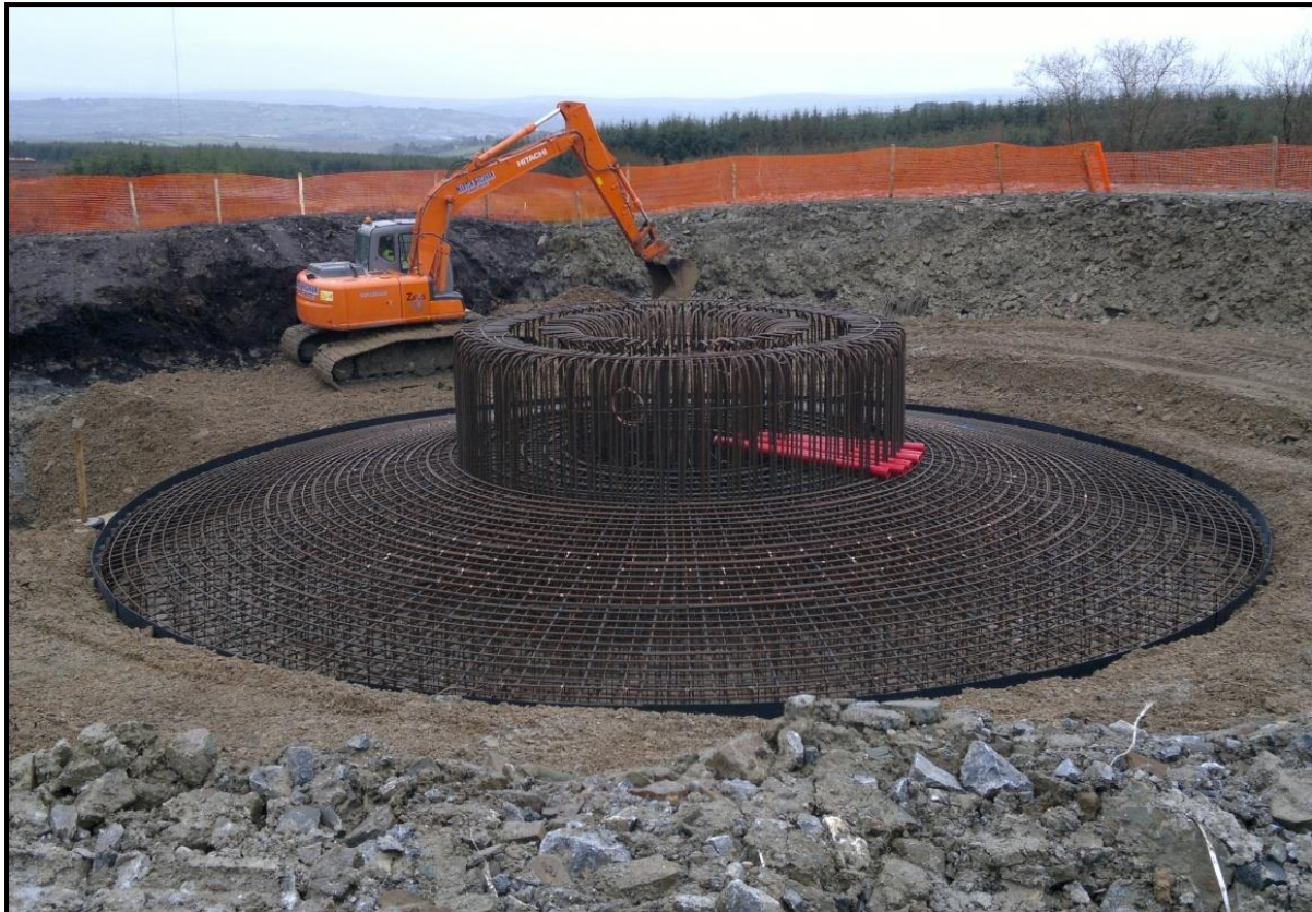
Plate 9. Typical construction of a wind turbine base.
